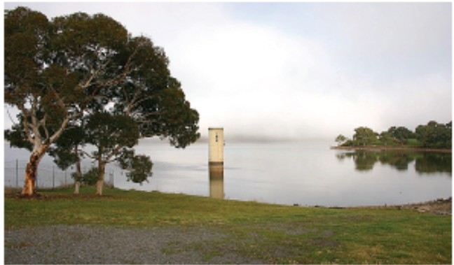
Tullaroop Reservoir tower
