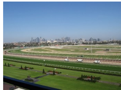
View from top of new members' grandstand
