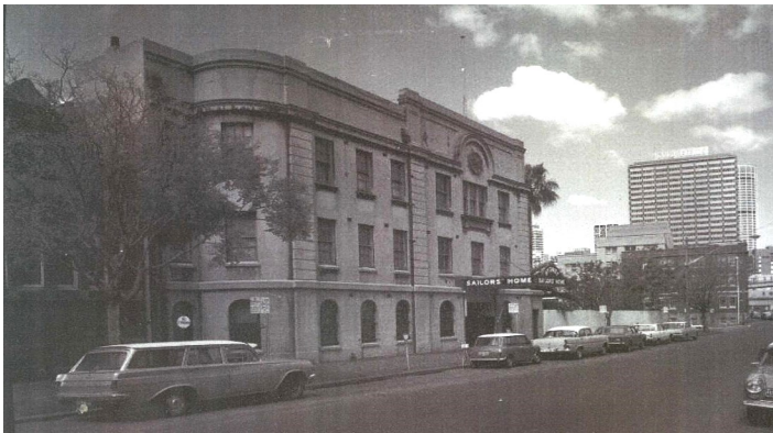
Former Sailors Home 106-108 George Street. Photo taken on 1st January 1970 by Tim Collis-Bird. Photo credit: Sydney Harbour Foreshore Authority
