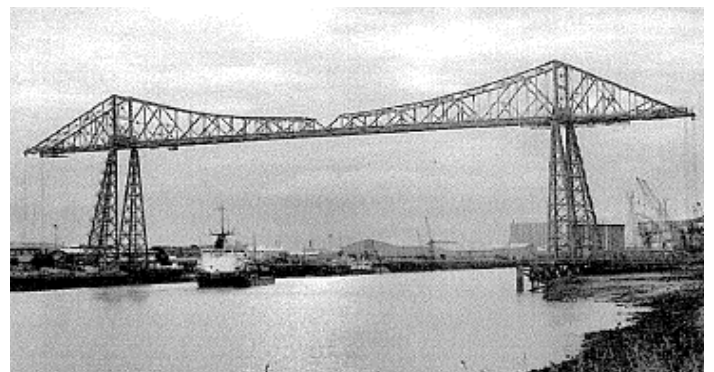
Transporter Bridge (also known as a Ferry Bridge) over the River Tees. It's a movable bridge which carries a segment of roadway. This one opened in 1911. There are a few left in the world, Another is in Newport, Wales.
