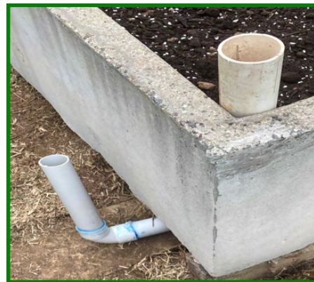
Water overflow pipe on left and water fill Pipe on right—placed before adding
